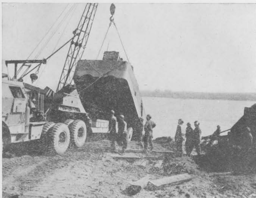
LCM BEING LAUNCHED BY A CRANE
