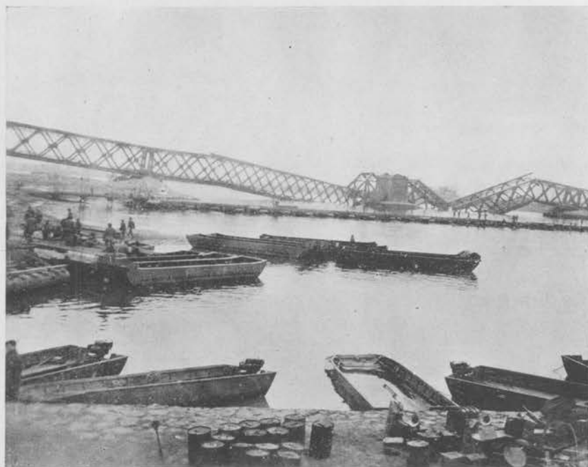
FOUR BOAT — THREE BAY PART UNDER CONSTRUCTION FOR 25-TON PONTON BRIDGE, WESEL
