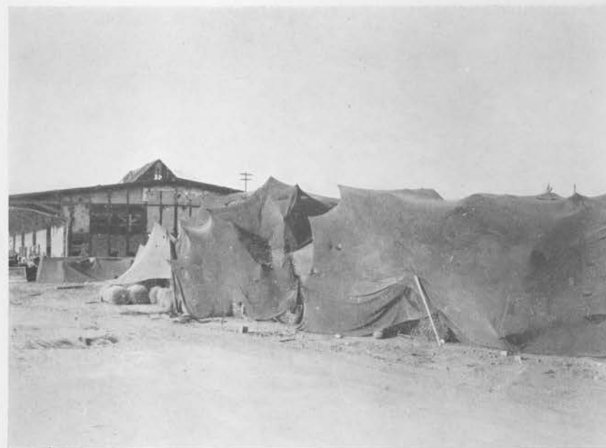
SHRIMP NETS PROPPED WITH POLES USED TO COVER RIVER CROSSING MATERIALS, 1143D ENGINEER COMBAT GROUP BRIDGE PARK
