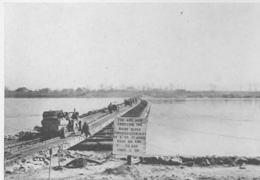
COMPLETED M2 TREADWAY BRIDGE AT WALLACH
