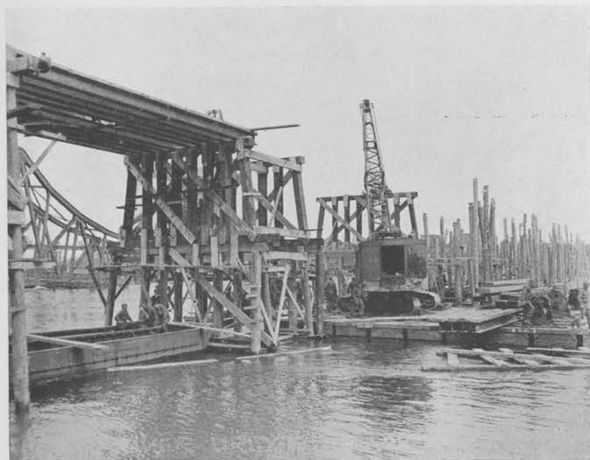
CRANE MOUNTED ON NL PONTON BARGE PLACING PREFABRICATED BENT ON PILING
