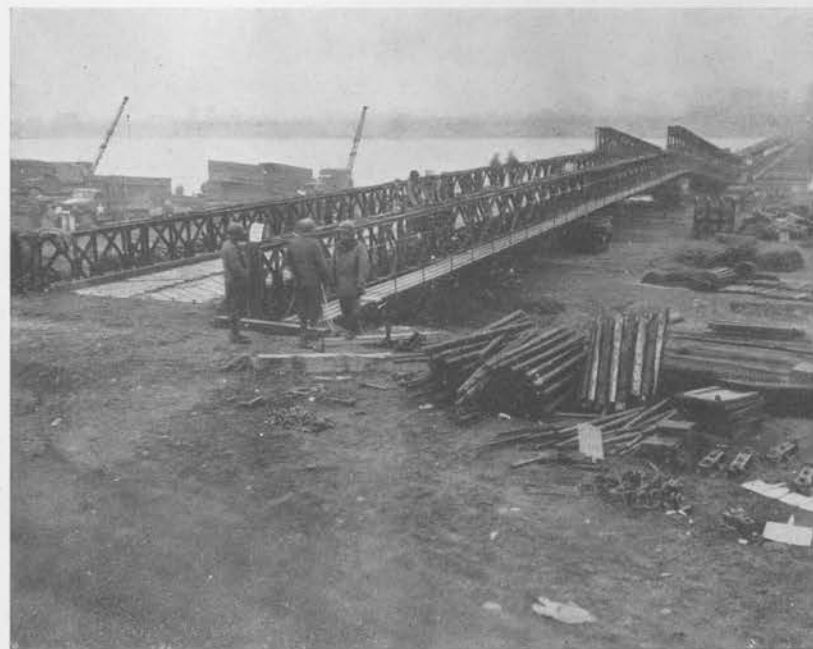
WEST APPROACH TO CLASS 40 BAILEY BRIDGE AT WESEL
