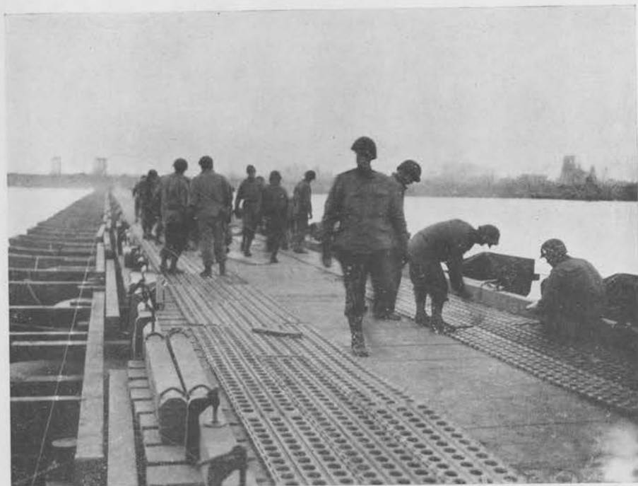
PIERCED PLANK USED FOR TREADS
