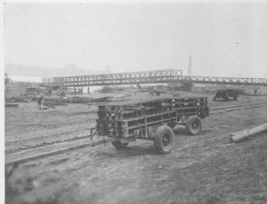
NEAR SHORE LANDING BAY IN PLACE, BAILEY BRIDGE NO. 3
