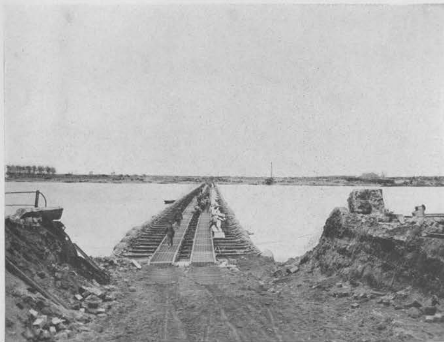
FAR SHORE APPROACH, TREADWAY BRIDGE AT WESEL
