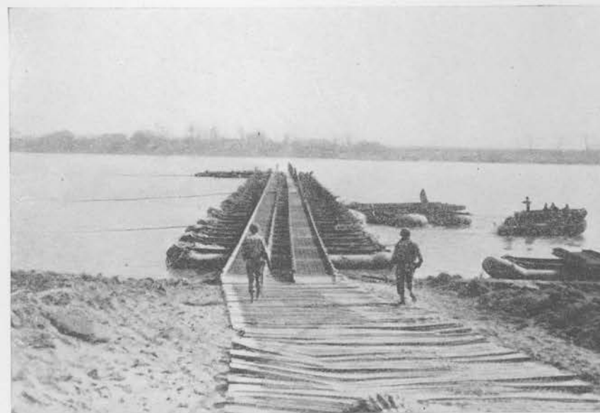
M2 TREADWAY BRIDGE UNDER CONSTRUCTION AT WALLACH. NOTE THE PREFABRICATED ROADWAY
