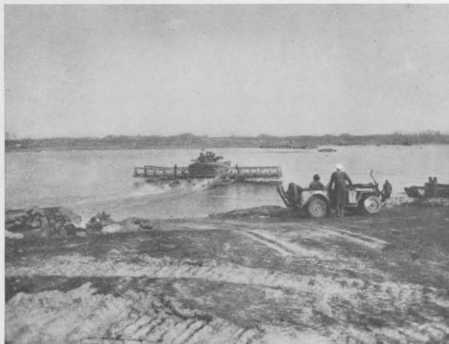
MEDIUM TANK BEING CARRIED TO FAR SHORE ON CLASS 40 BAILEY RAFT. OFFICER WEARING THE WHITE HELMET IS "BEACHMASTER"
