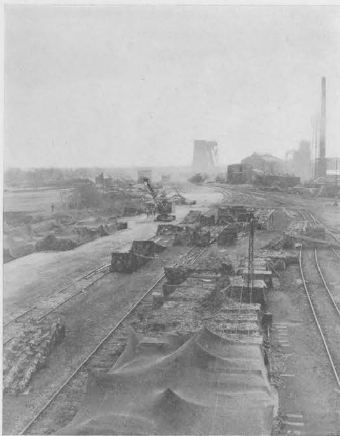
LINTFORT BRIDGE PARK. NOTE DIFFERENT TYPE NETS USED
