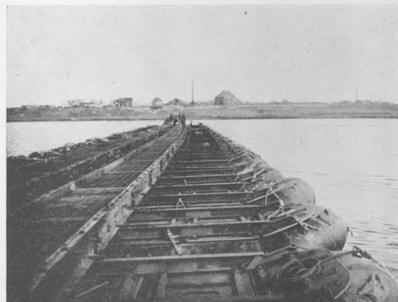
M2 TREADWAY BRIDGE AT MILCHPLATZ UNDER CONSTRUCTION
