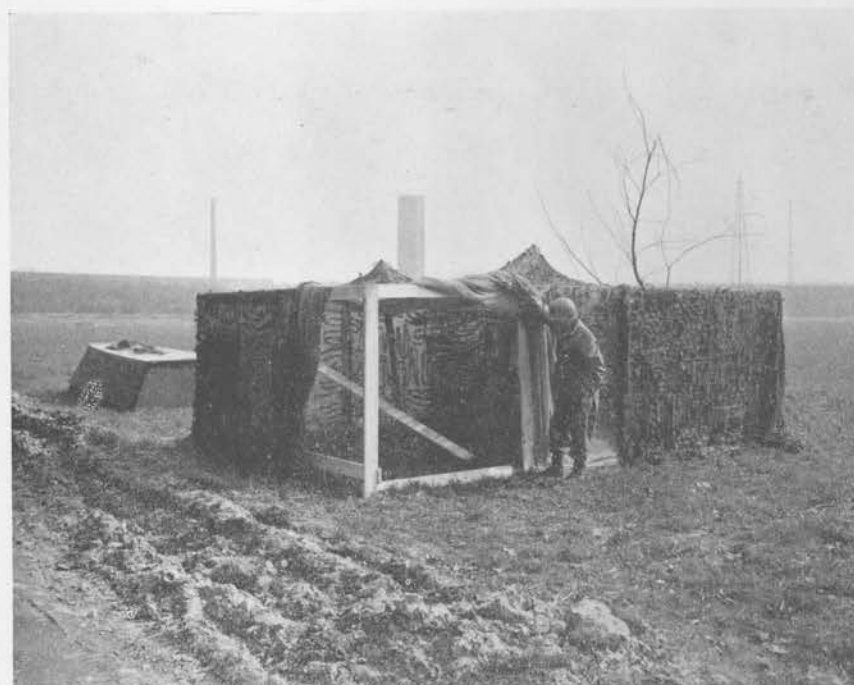
DECOY STACK OF SIMULATED BRIDGING MATERIALS. NOTE DUMMY ASSAULT BOAT IN BACKGROUND
