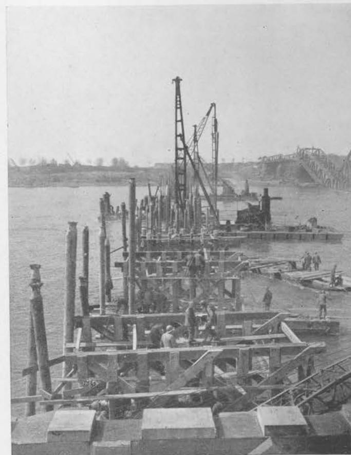
RHINE RIVER FIXED BRIDGE UNDER CONSTRUCTION. NOTE DEMOLISHED HIGHWAY BRIDGE IN BACKGROUND
