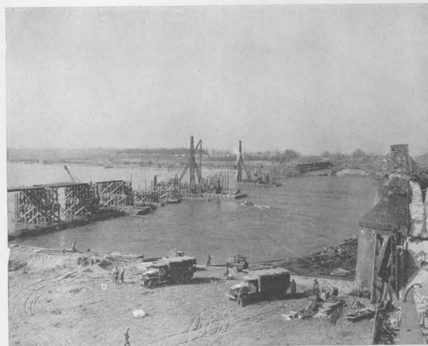
DRIVING PILES FOR THE RHINE RIVER BRIDGE
