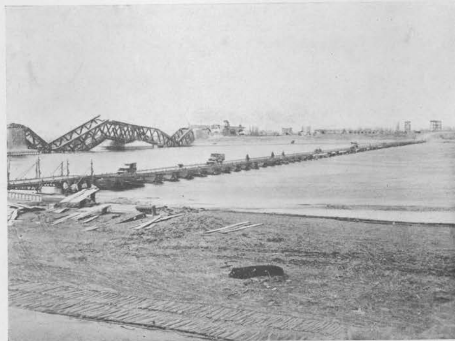
COMPLETED 25-TON BRIDGE CARRYING TRAFFIC AT WESEL
