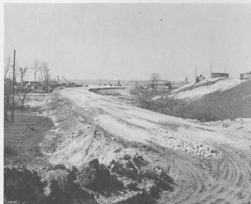
CONNECTING ROAD BETWEEN RHINE AND LIPPE BRIDGES NEARING COMPLETION
