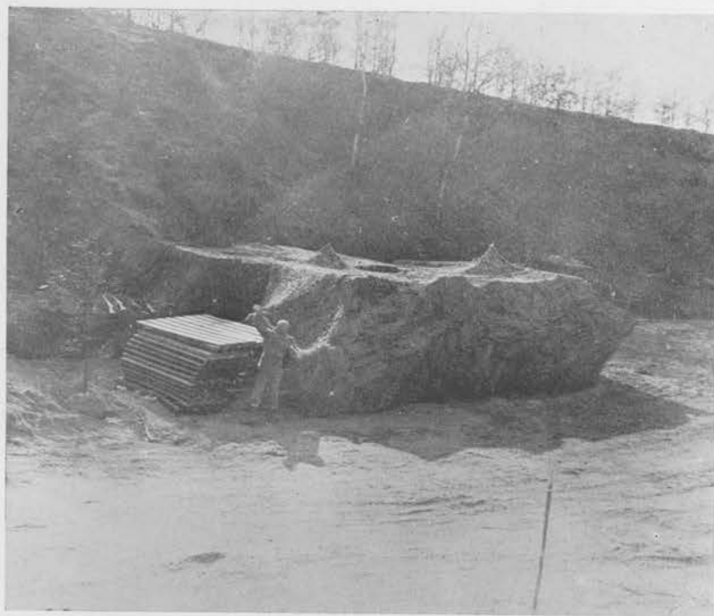
BRIDGING MATERIALS BEING CAMOUFLAGED, 1117TH ENGINEER COMBAT GROUP BRIDGE PARK
