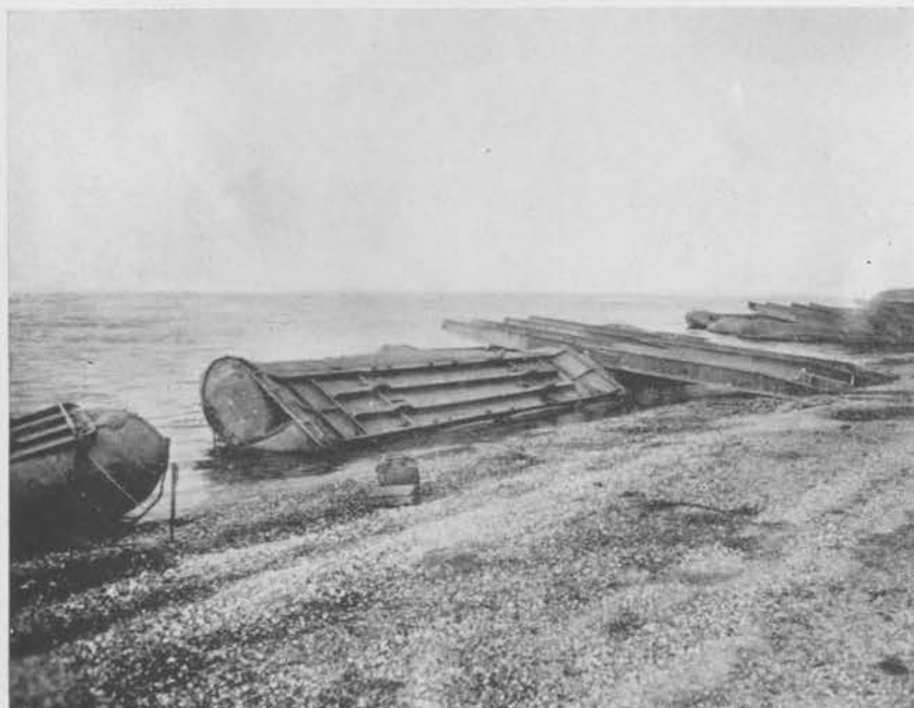
DAMAGED FLOATS CAUSED BY CLASS 40 BAILEY RAFT DRIFTING INTO M2 TREADWAY BRIDGE AT WALLACH
