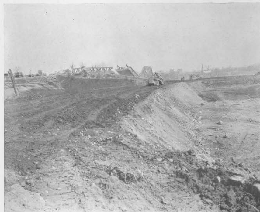
FILL NEARING COMPLETION — WEST APPROACH, RHINE RIVER FIXED BRIDGE
