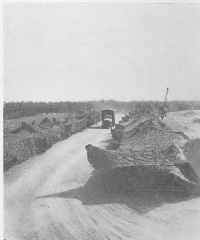
BRIDGING MATERIALS STACKED ALONG EACH SIDE OF ROAD AND CAMOUFLAGED 1142d ENGINEER COMBAT GROUP BRIDGE PARK
