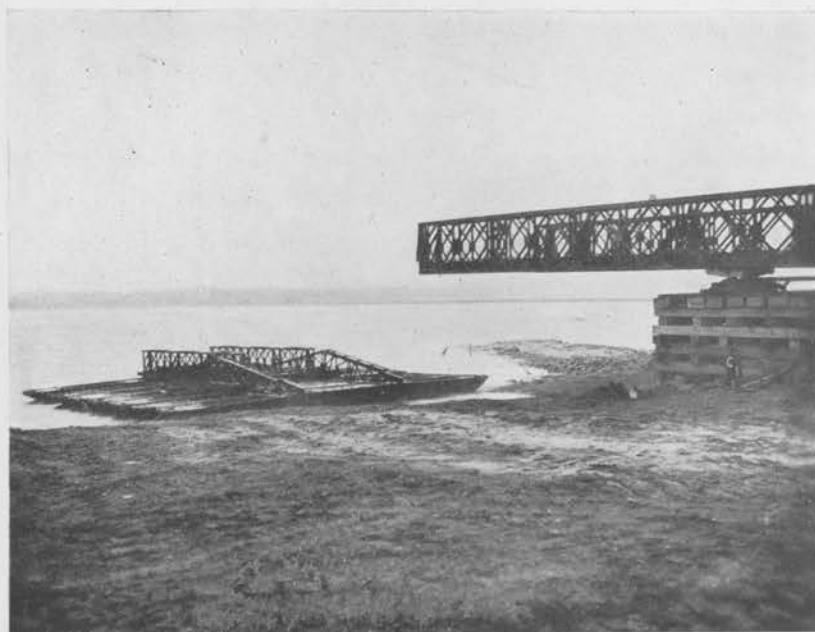
NEAR SHORE LANDING BAY OF BAILEY BRIDGE NO. 1 BEING LAUNCHED. NOTE LANDING BAY PIER BROUGHT INSHORE; ALSO TIMBER CRIB PIER ON BANK
