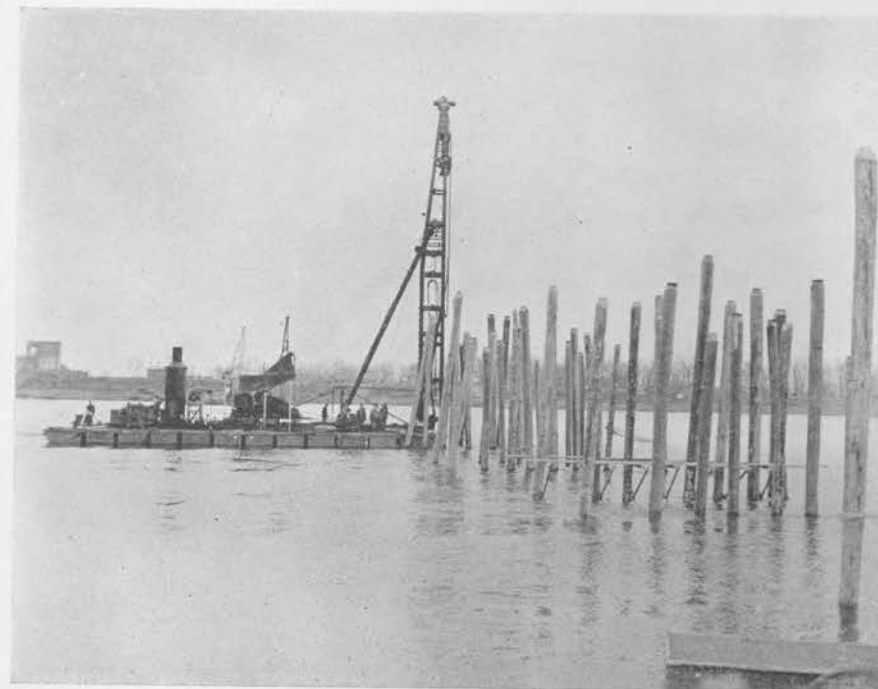
SKID MOUNTED RIG WITH 66-FOOT LEADS AND VULCAN STEAM HAMMER MOUNTED ON NL PONTOON BARGE
