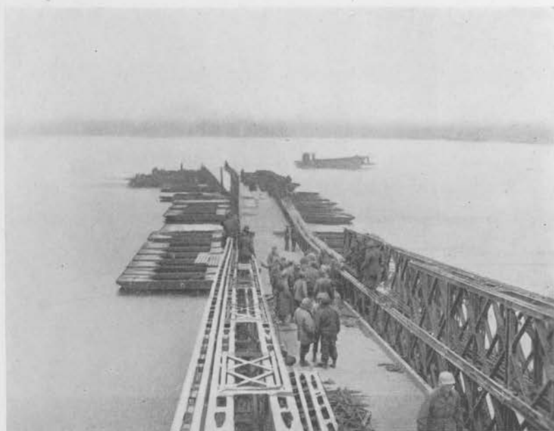
ADDING SECOND STORY TO NEAR SHORE LANDING BAY, BAILEY BRIDGE NO. 1
