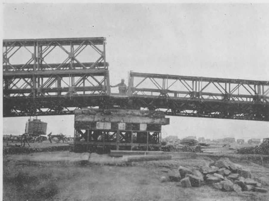
LANDING BAY AND FIXED SPAN RESTING ON STEEL CRIB PIER AT NEAR SHORE END OF BAILEY BRIDGE NO. 3
