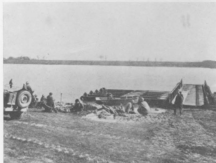
CLASS 40 BAILEY RAFT ANCHORED TO NEAR SHORE AT BLUE BEACH
