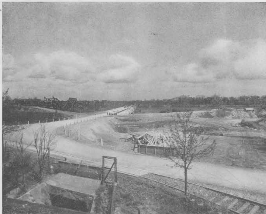
COMPLETED WEST APPROACH RHINE RIVER FIXED BRIDGE
