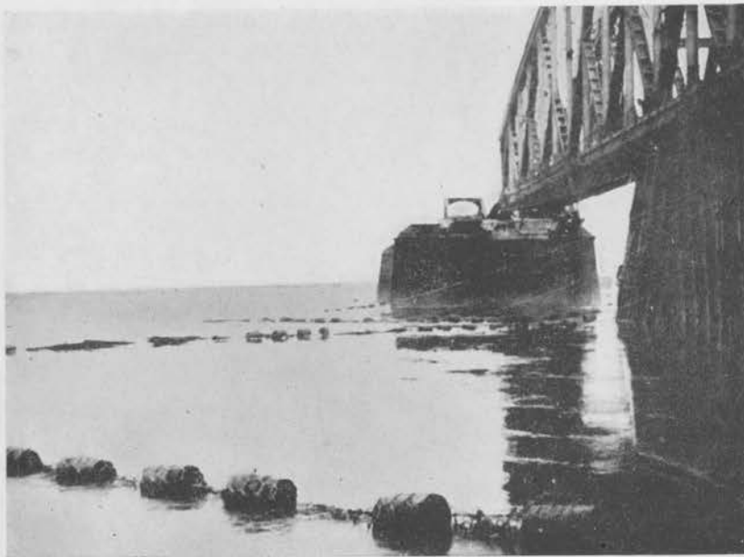
GROMMET TYPE NET BOOM INSTALLED, VICINITY OF HOMBERG
