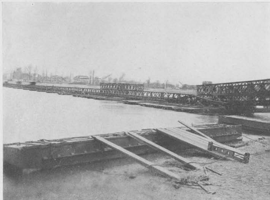
COMPLETED BAILEY BRIDGE AT WESEL. NOTE SLIDING BAY TOWARD MIDSTREAM
