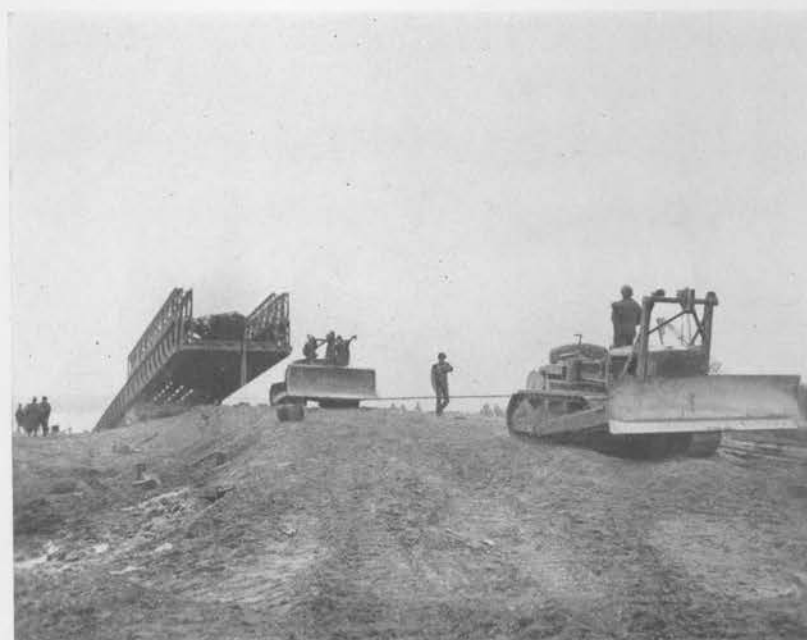
LAUNCHING NEAR SHORE LANDING BAY OF BAILEY BRIDGE NO. 1 WITH AID OF BULLDOZERS
