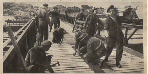
THREE HOURS LATER: The Last Section of the Bridge is Got Into Place
