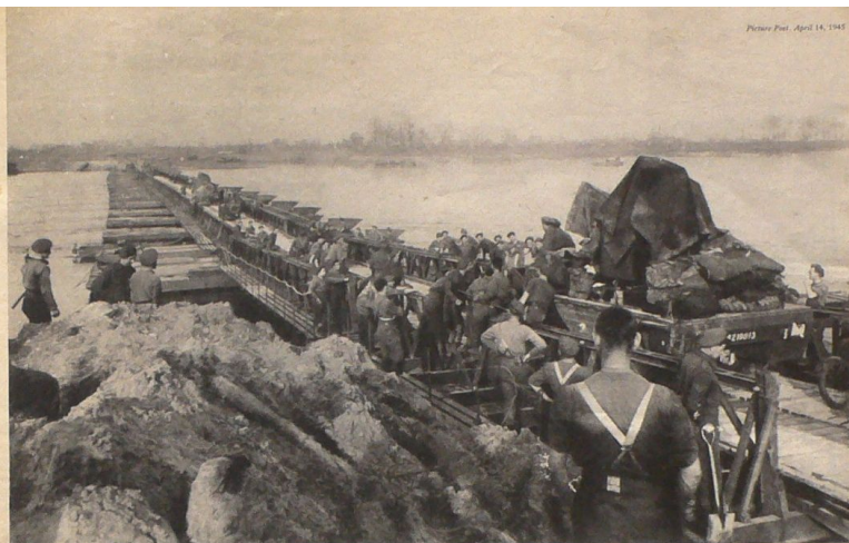
14.30 HOURS ON D-PLUS ONE: The First Pontoon Bridge Across the Rhine is Opened for Heavy Traffic. The job has been completed nearly half a day ahead of schedule. The first vehicles to go across, after the chief engineer has made his final check, are mobile guns for the anti-aircraft defences of the bridge on the eastern bank of the river.
